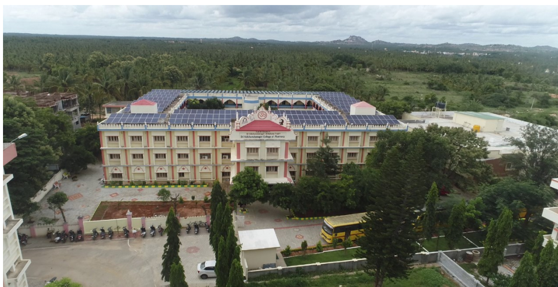
Solar panels on roof top
