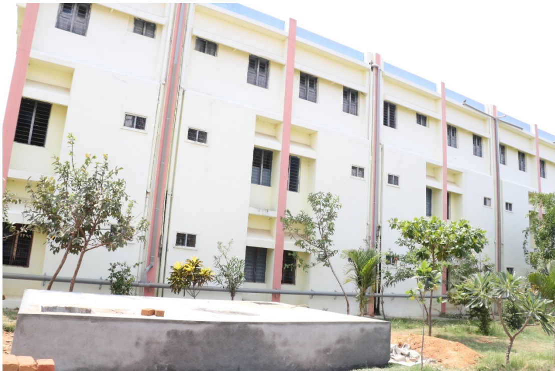
Rain water harvesting tank
