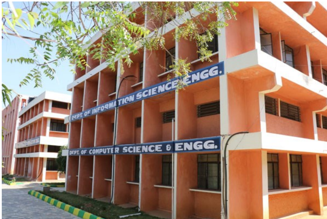
A passive architectural design with clerestory window for classrooms
