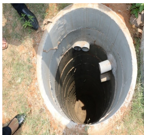
Rain water collection tank.
