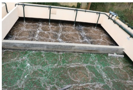
MBBR unit in Sewage Treatment Plant. Screening unit in Sewage Treatment Plant.
