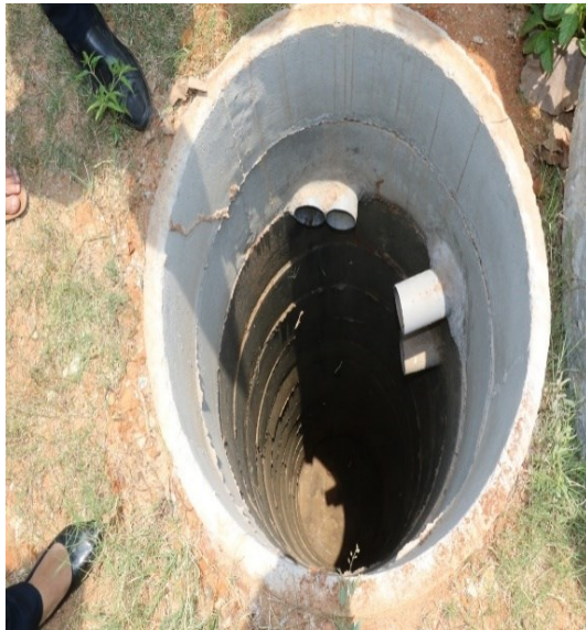
Rain water Recharge Pit
