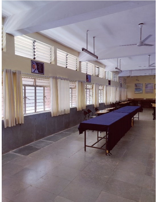
A passive architectural design with clerestory window for classrooms
