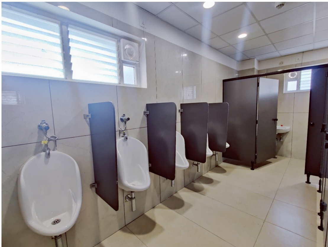
Urinals with auto release flush valve
