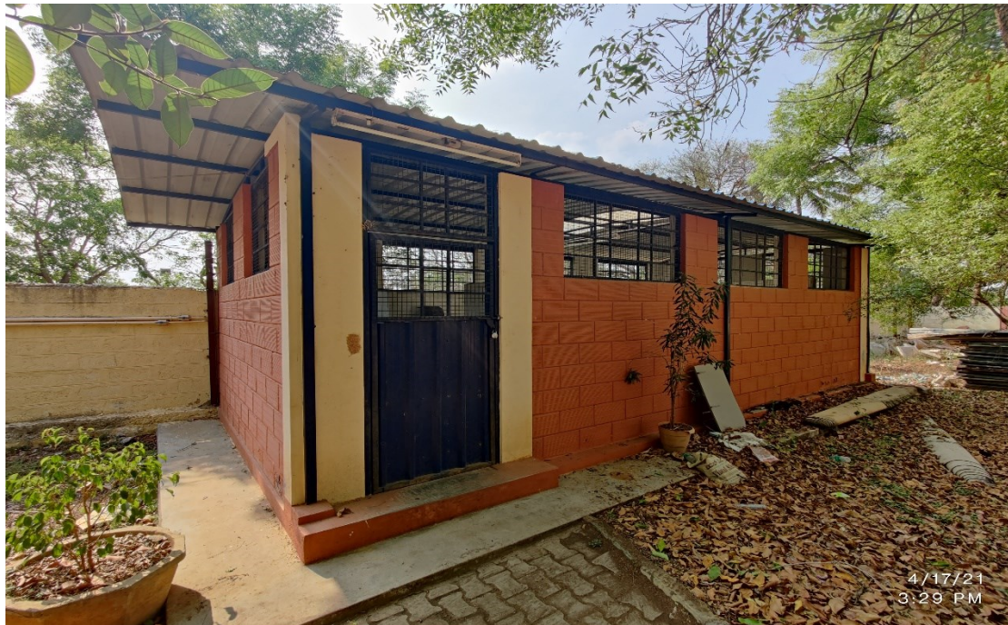
Treated waste water used for flushing.
