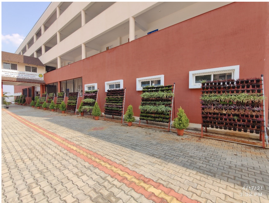
Vertical greenery systems, used as a strategy for urban heat island mitigation.
