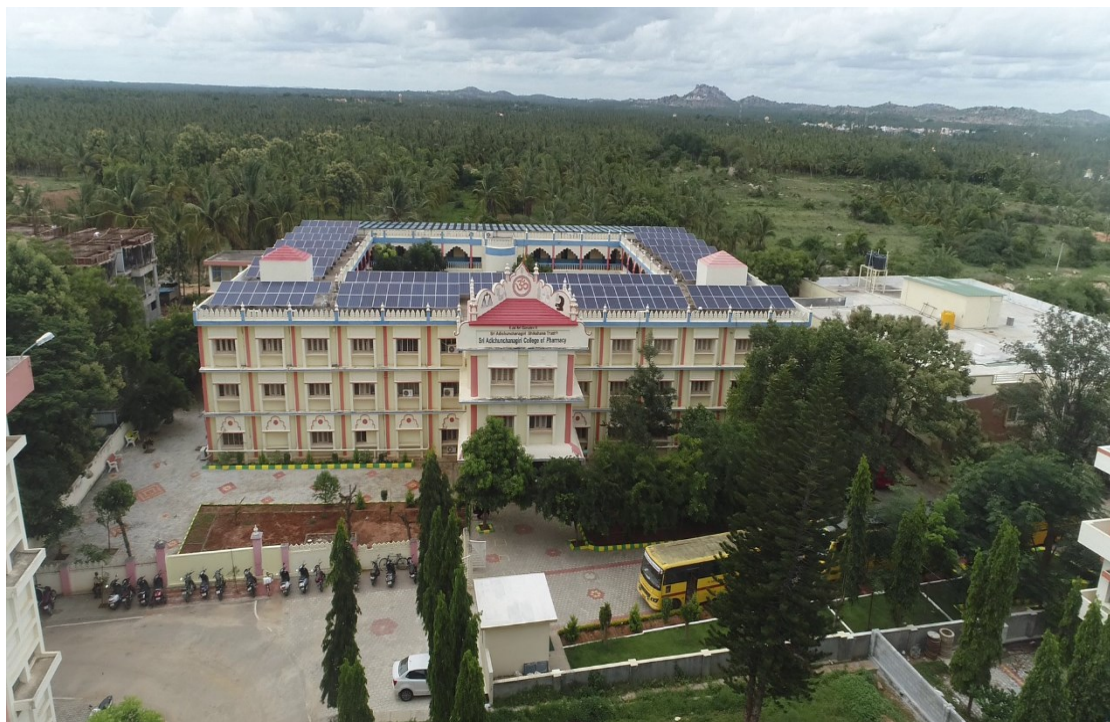
Solar panels on roof top
