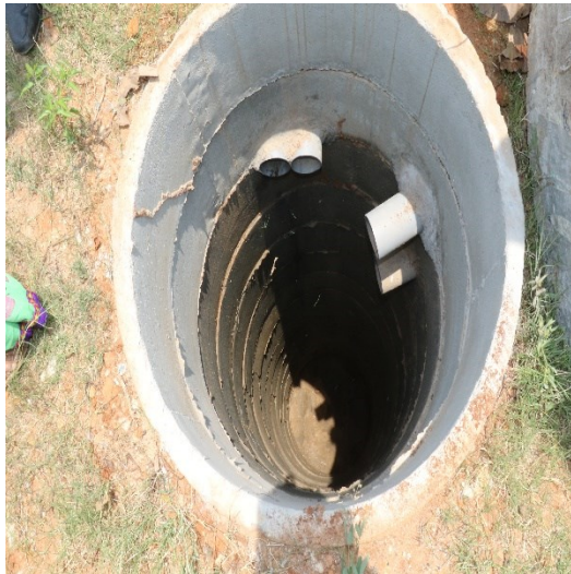
Rain water Recharge Pit
