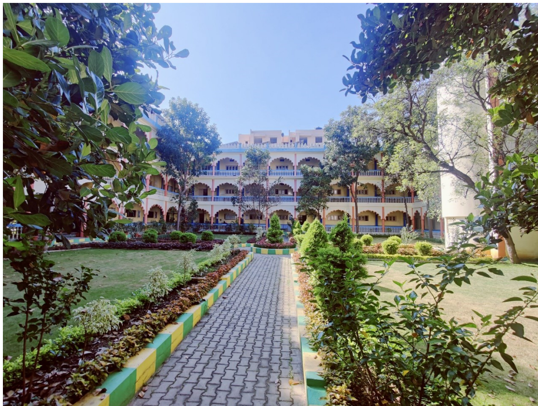
Vegetation inside and outside the building to purify air
