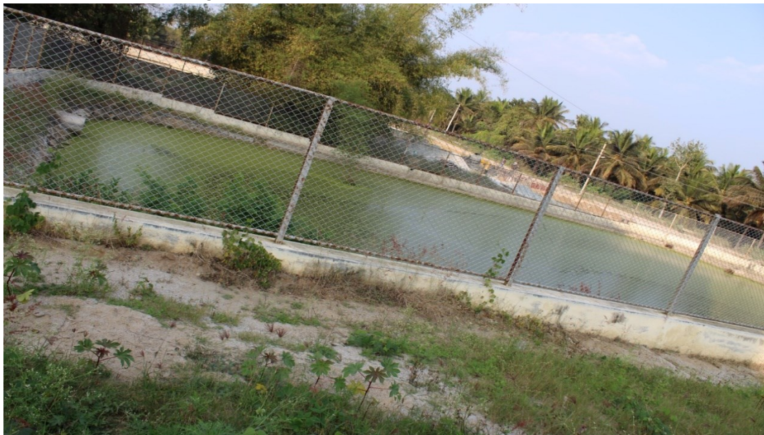
Rain water collection tank.
